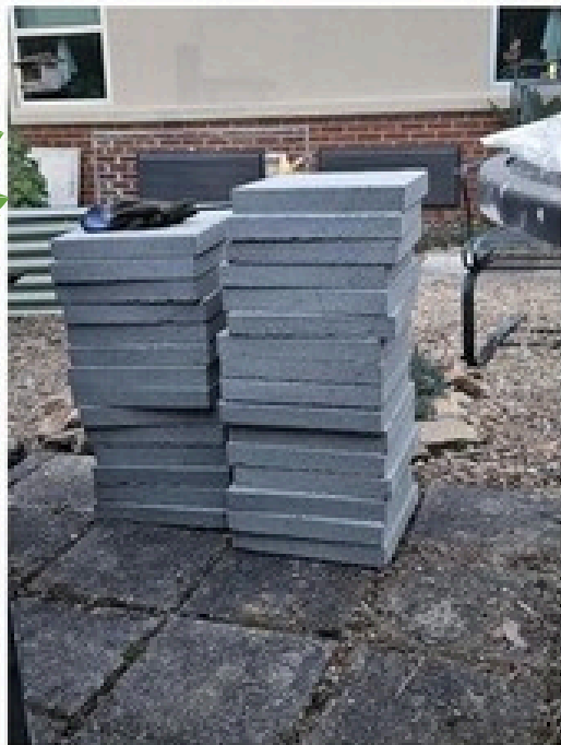
Blocks for patio extension
